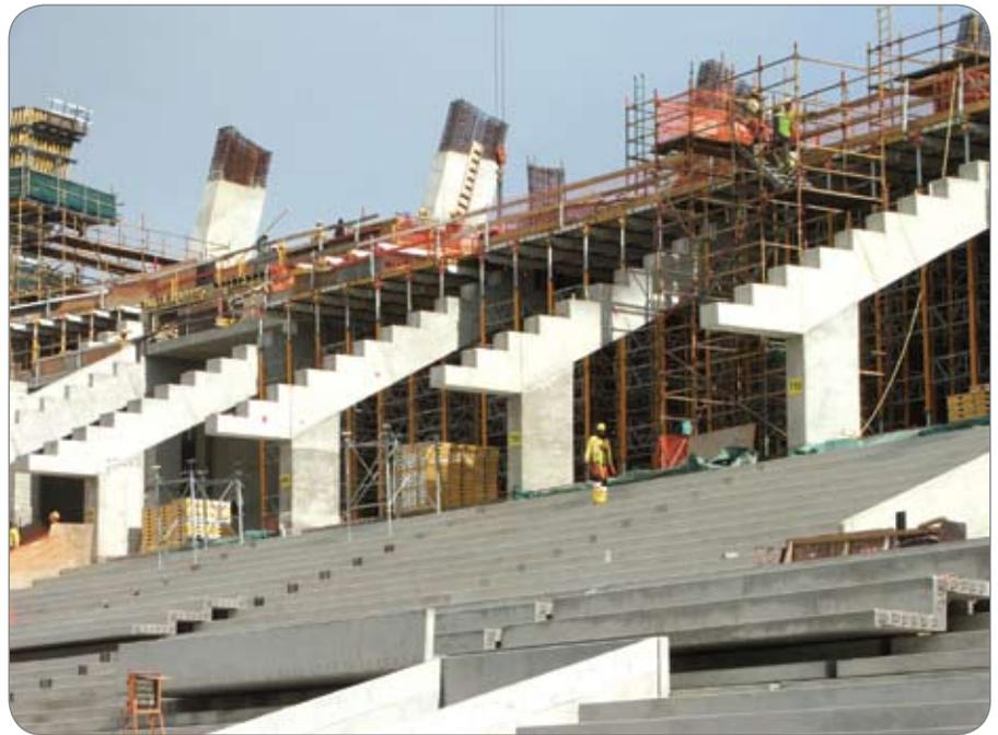
Fig. 7: Raked beams on which the 20 ton precast seating elements will rest.
