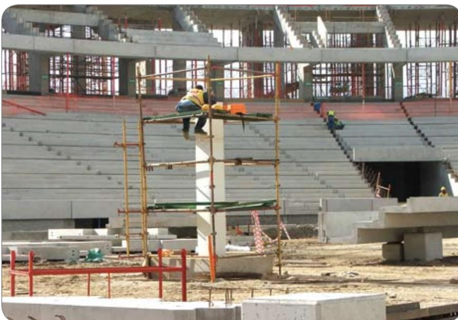
Fig. 6: Checking the placing position of the precast seating elements from a 4 m high pillar on the future pitch.
